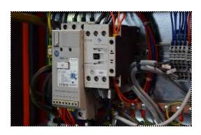
Motor **soft-starter** allows a reduction of the load and torque in the power train and electrical current surge of the motor during start-up.
